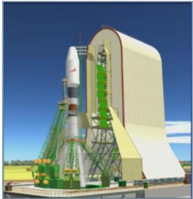
Fig. 2. Mobile gantry intended for Soyuz-ST servicing
