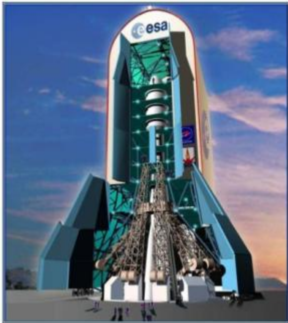
Fig. 2. Mobile gantry intended for Soyuz-ST servicing
